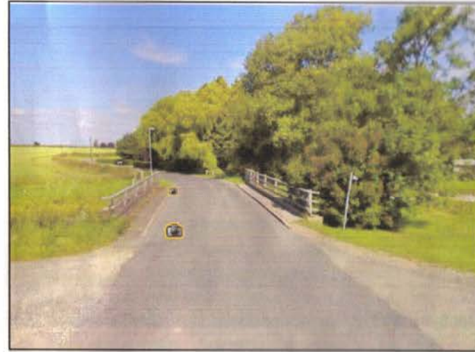
Bridge over canal 2010 *
