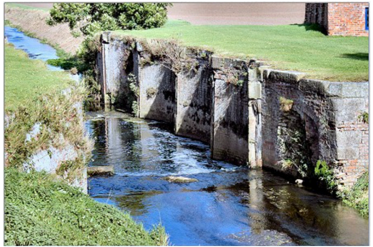
Alvingham Lock, barrel-shaped design
