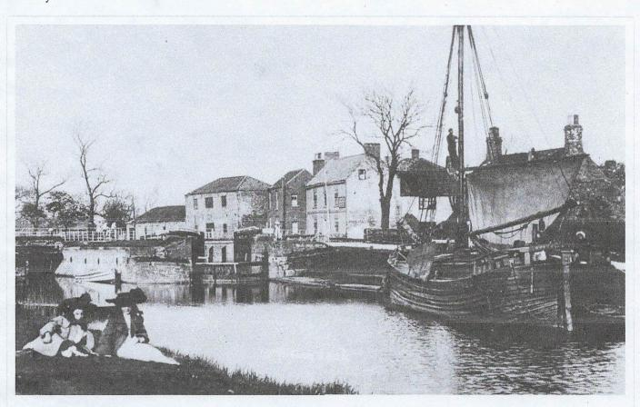
This image shows an empty *Reliance* moored above Tetney Lock waiting for its chance to continue through into the Humber Estuary. Notice the outer sea gates are closed as the lock was designed so it could be navigated, no matter if the water level of the Humber was above or below that of the canal.
