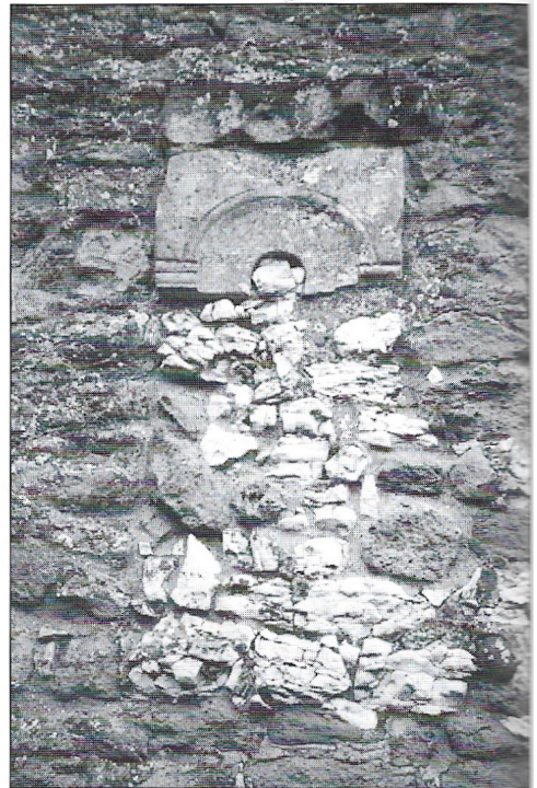
The remains of a small Saxon window on the north wall of St. Mary's Church. (Photo: the author, 2000).
