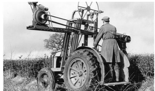
Figure 7: Machine with reciprocating blade cutters that somewhat decreased hedge-cutting times
